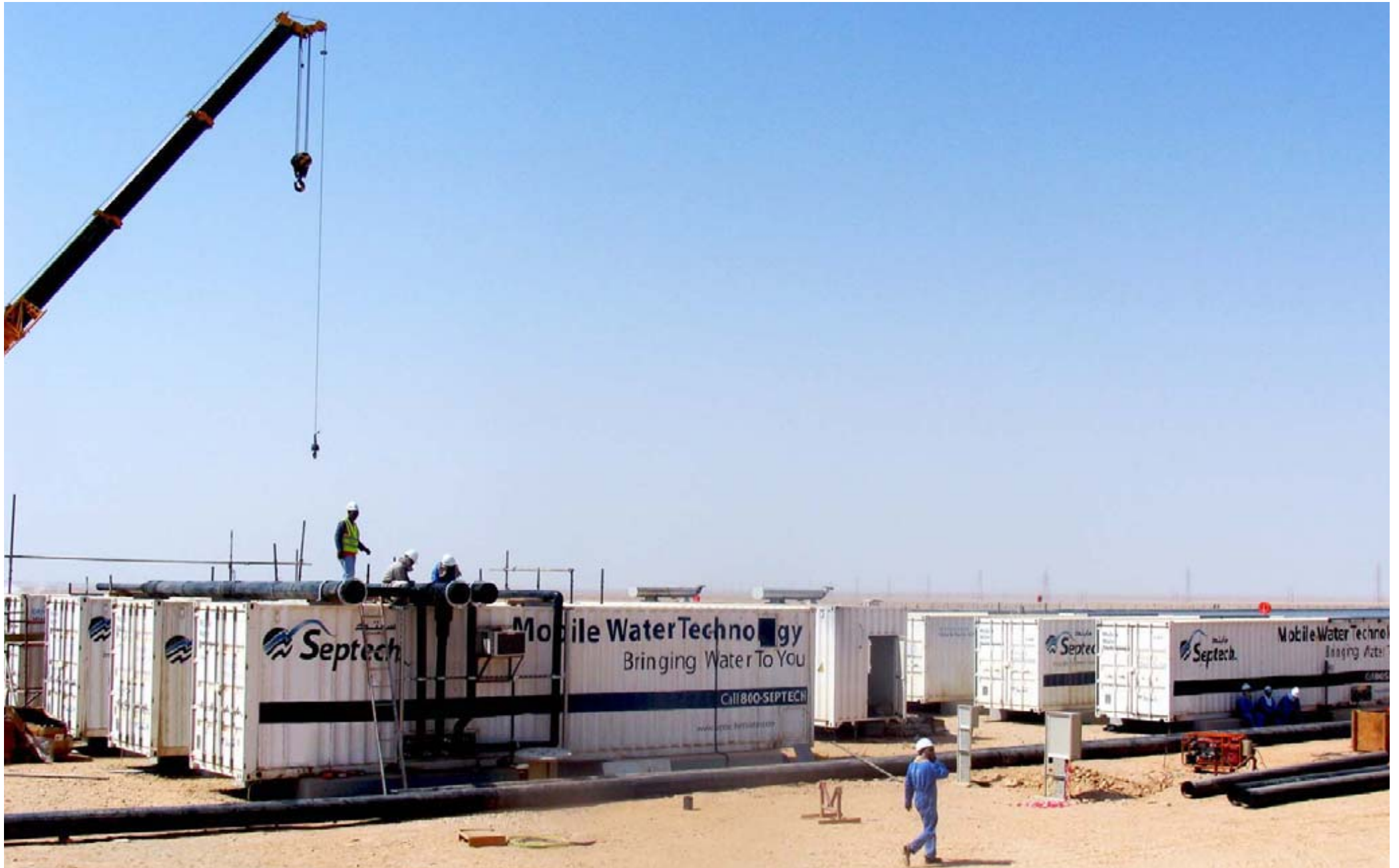
Septech Mobile Water Treatment Plant, Mukhaizna
