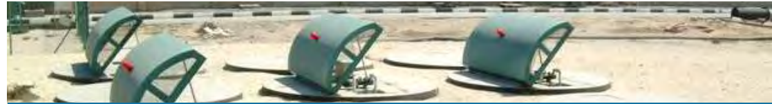
Underground Trickling Biofilters
