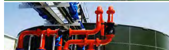
Extended Aeration Plant(Capitox)
